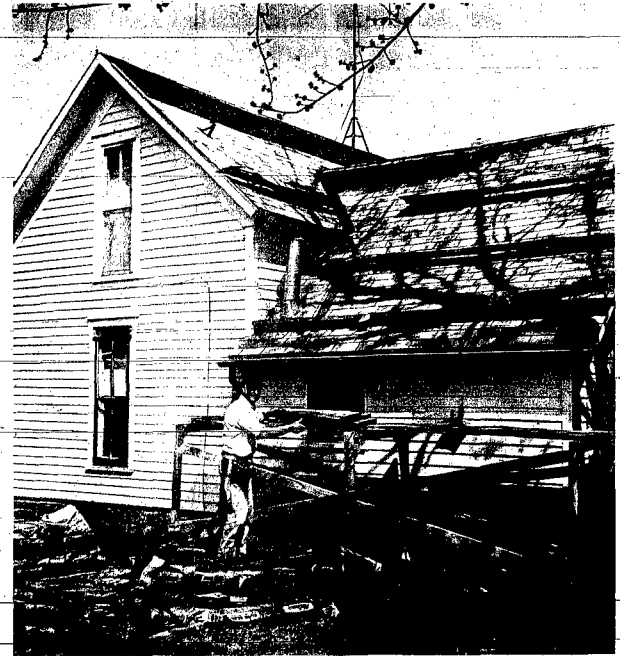
Elvis Olson, Wakefield, works at a new roofing job for the Mrs. Harry Swinney residence on Third and Blaine Streets.
